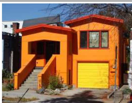
Figure 2-1 Typical house with cripple walls.
