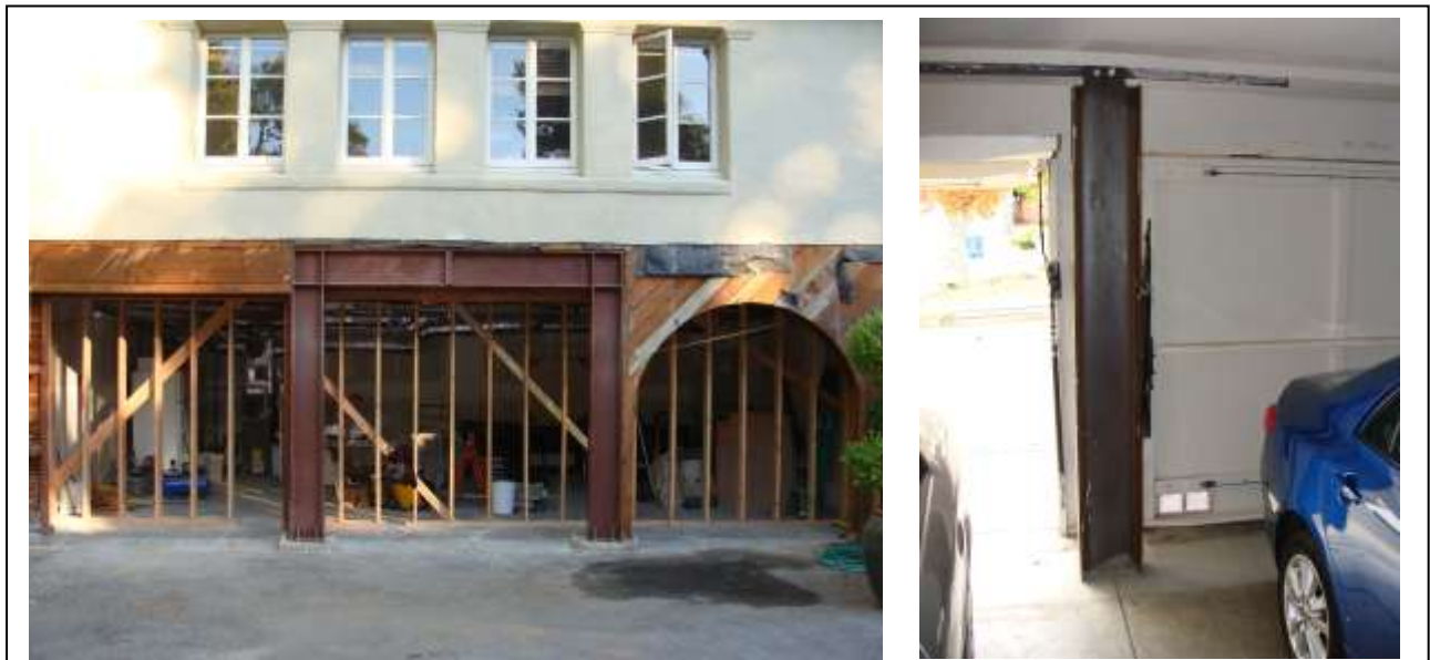
Figure 4-2 Two ways to strengthen a soft-story.
