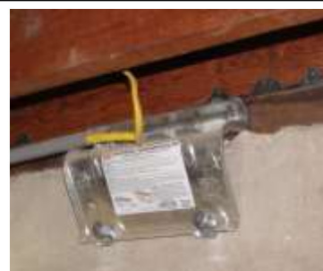
Figure 3-4 A Simpson “UFP10” used where bolt holes could not be drilled from above (yellow electrical cable and gray conduit to left are not related to the connector).
