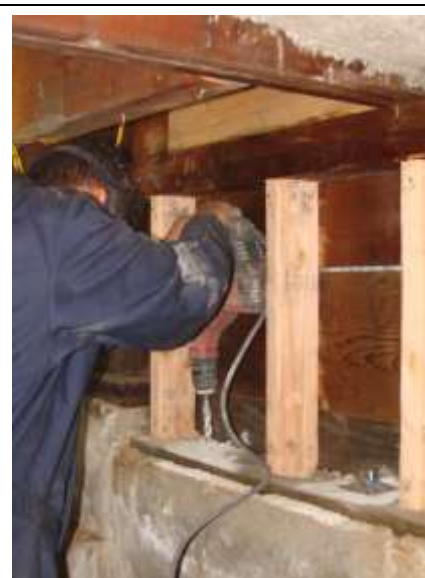
Figure 3-3 Retrofit bolt installation at a cripple wall.
