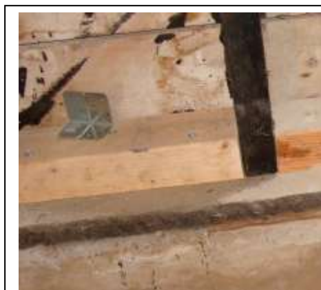
Figure 3-8 Mudsill blocks connected with structural screws.
